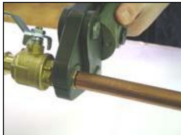
H. Start the pressing process and hold the trigger until the jaw has engaged the fitting.
