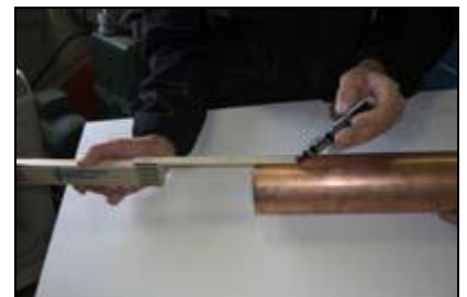
C. Mark proper insertion depth: 2.125" for 2-1/2" and 3" valves, 2.5" for 4" valves. Improper insertion depth may result in an improper seal.
